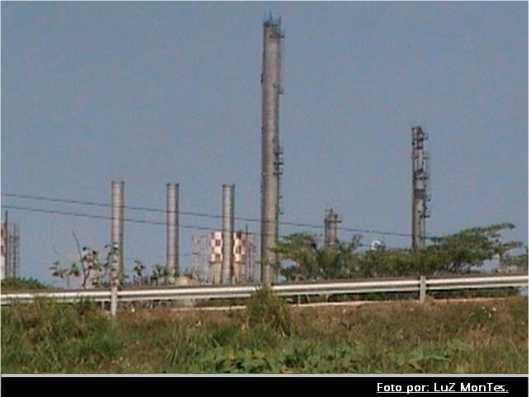
View from the sampling site at the petrochemical complex.
